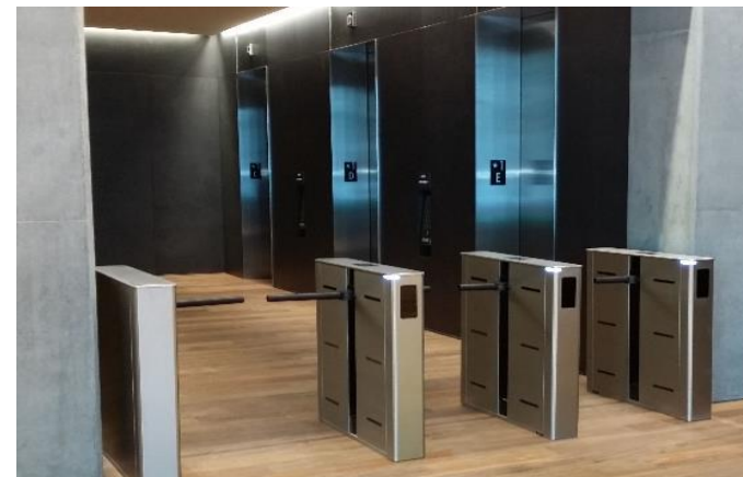
Elevator hall of parking lot
